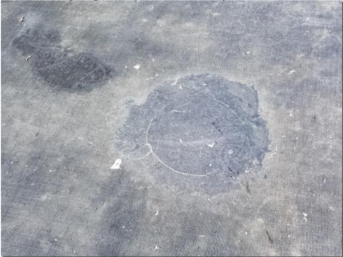
Here is what last years geotextile patch looked like this year:
